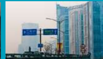
Next to Airport Expressway
